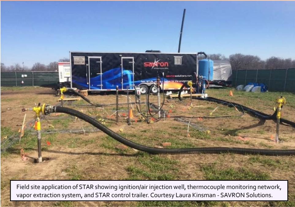
Field site application of STAR showing ignition/air injection well, thermocouple monitoring network, vapor extraction system, and STAR control trailer. Courtesy Laura Kinsman - SAVRON Solutions.
